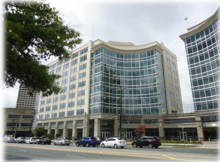
Figure 1: Exterior View from Across Rockville Pike
